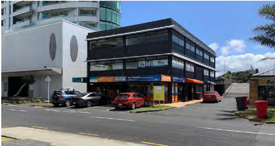
Figure 4: Street Frontage of the Subject Site
